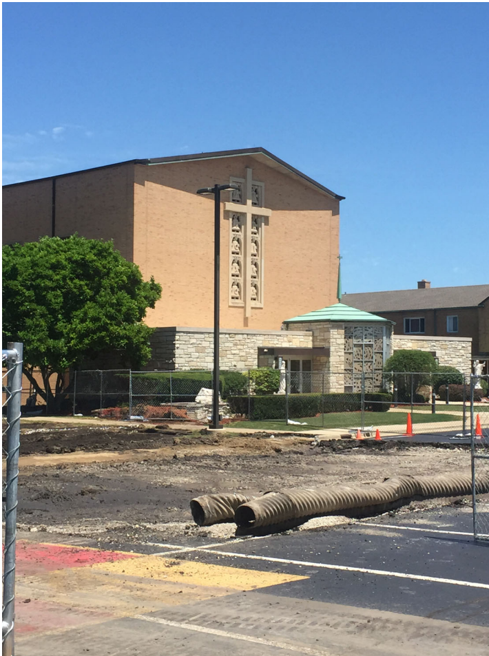
Construction on our new Parish Center has begun!
