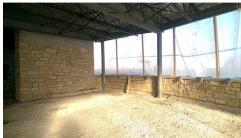
Inside the meeting rooms
