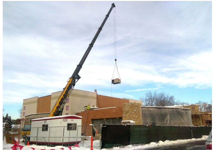
Installation of the heating unit.
