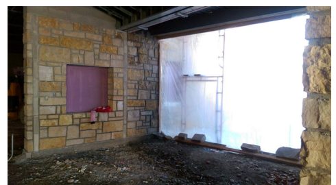
A view of the entrance to the new building
