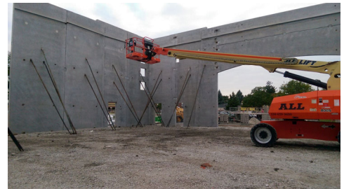
The walls going up in October
